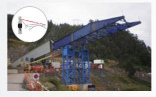
This type of monitoring is used to control the positioning of mobile elements which have to be placed in a specific place as set out and detailed in the project plans. Bridge launching is a clear example of dynamic monitoring.
