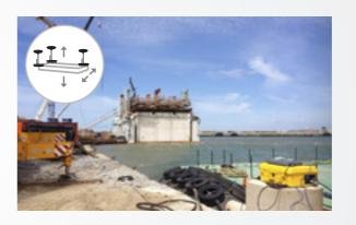
This type of monitoring is used for controlling the placement of concrete blocks and for verifying displacement of structures. A good example of this kind of monitoring is the sinking of concrete caisson blocks in maritime works, or the close control of areas where there could possibly be structural movement.
