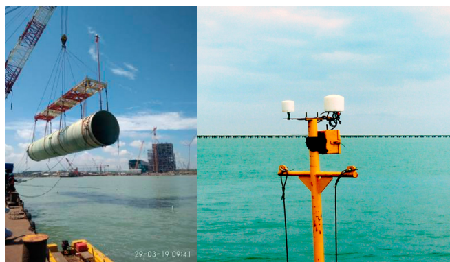
Figure 8 & 9: Version 1 (left) - Single RTK positioning of pipe, Version 2 (right) With heading capability
