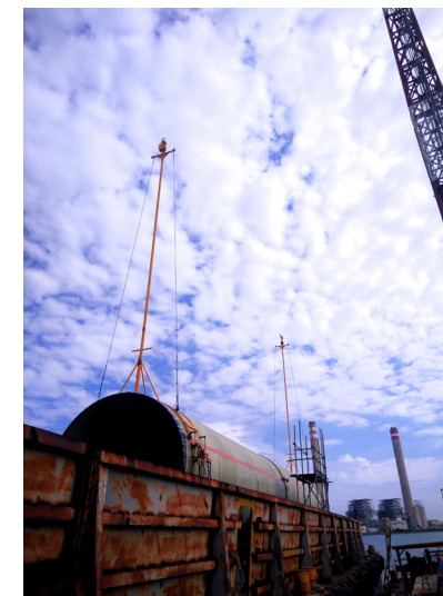
Figure 5: Prism and guide bar in the original method
