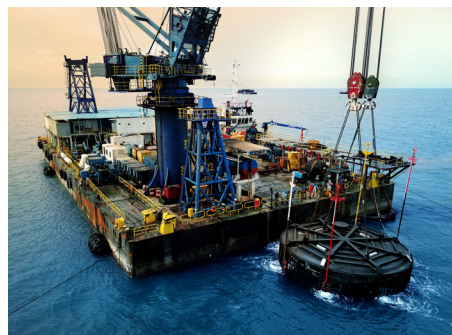
Figure 1: Clam shell dredger and marine construction operation
